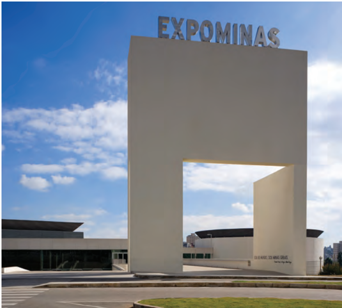
Facade of Expominas, Trade Fair and Expo Center.
